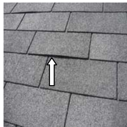
Shingle tabs not secure
